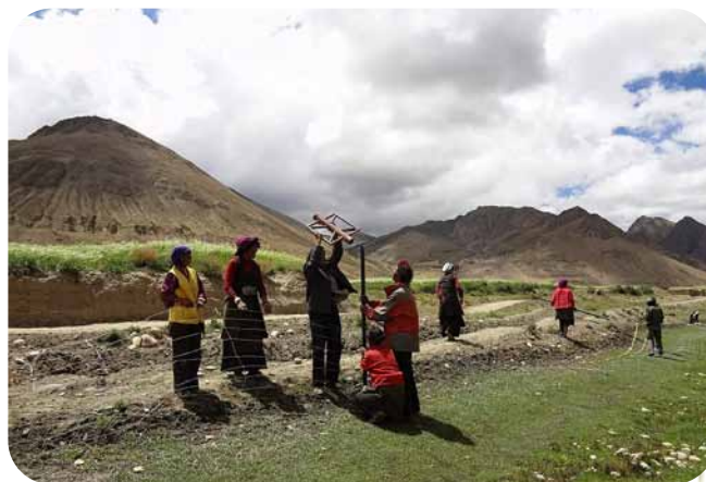
楚西村村民正在搭建湿地围栏 Villagers of Chuxi work on building wetland enclosures
